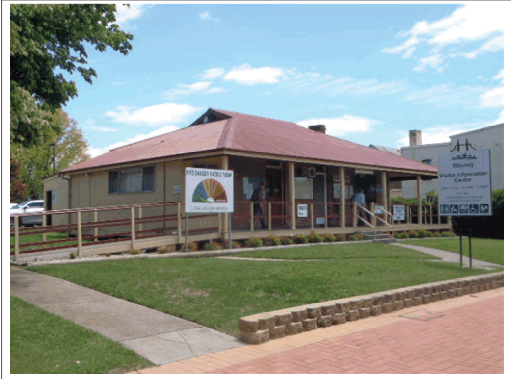
The Cottage, 97 Adelaide Street, Blayney NSW 2799
